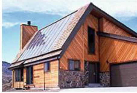
Fig. 9.6 A home using a liquid-based solar system for space and water heating. The solar units are environmentally friendly and can be installed on roof to blend with the architecture of a house [18, 26]
