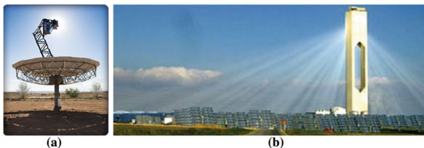
Fig. 6.17 a Stirling solar dish power production. b World's first commercial solar power tower located in Seville, Andalusia, Spain
