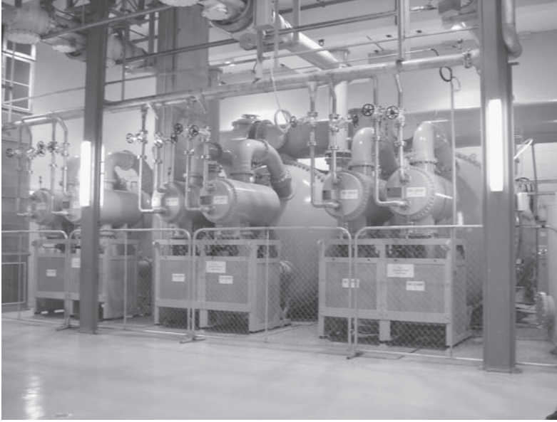
Haymarket substation (Australia)
