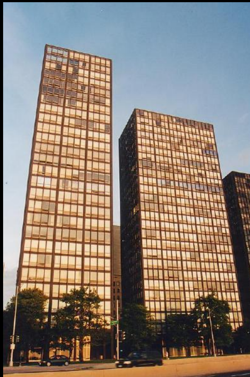
LAKE SHORE DRIVE APARTMANS, CHICAGO
