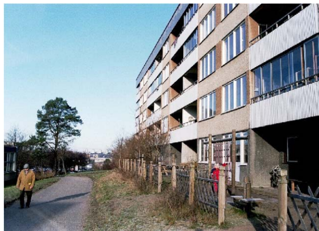
Fig. 3. Facade of the studied multi-dwelling house.
