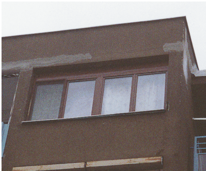
Figure 2. : A horizontal crack formed on the facade wall
