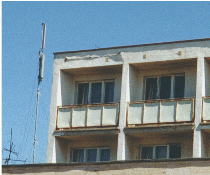
Figure 2. : A horizontal crack formed on the facade wall
