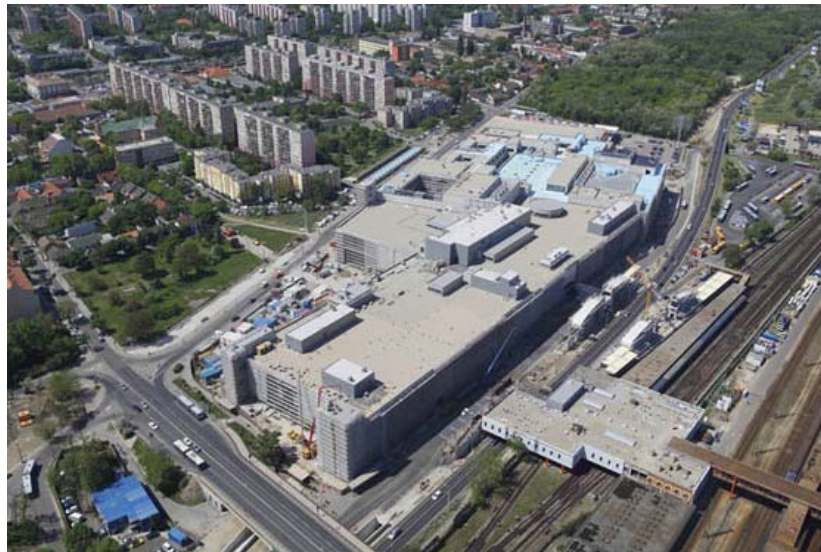
Fig. 4: The terminal after the refurbishment in 2011
