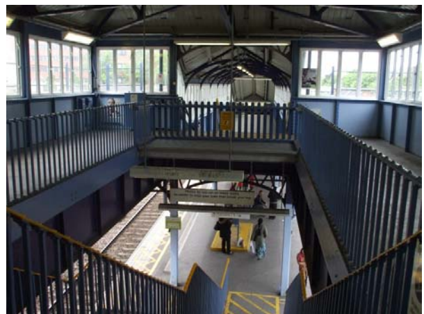
Views of walkway and stairs to platform 2/3. This design, allowing passengers to take two sets of stairs helps passenger flow during rush hour.
