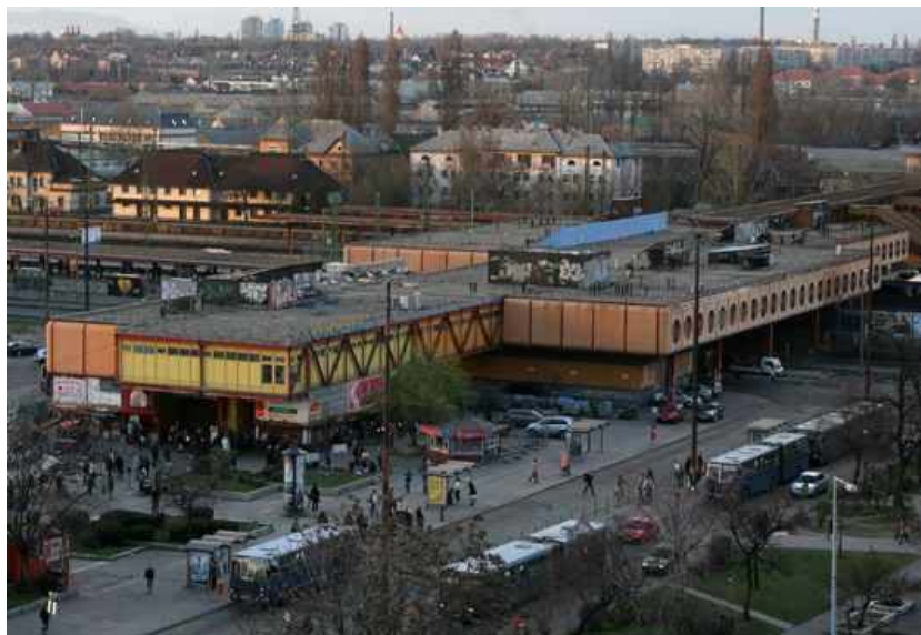
Fig. 3: The condition of the terminal, before the refurbishment, in the 2000's
