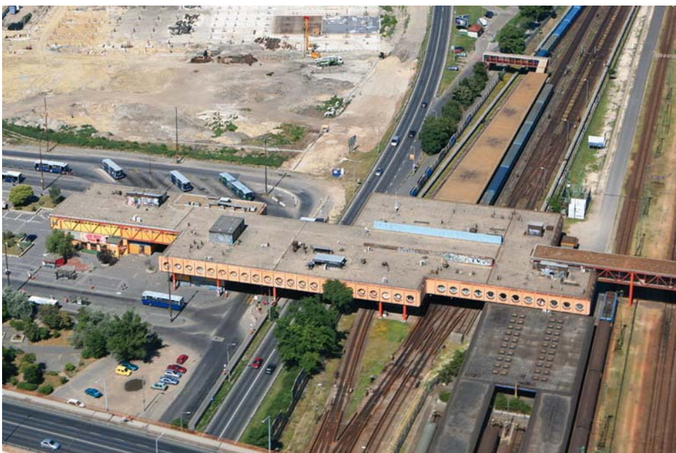
Figure 10: Aerial view of the terminal before the refurbishment (source: http://www.globalplaza.hu/hir/oktober-14-en-nyit-a-koki-terminal )
