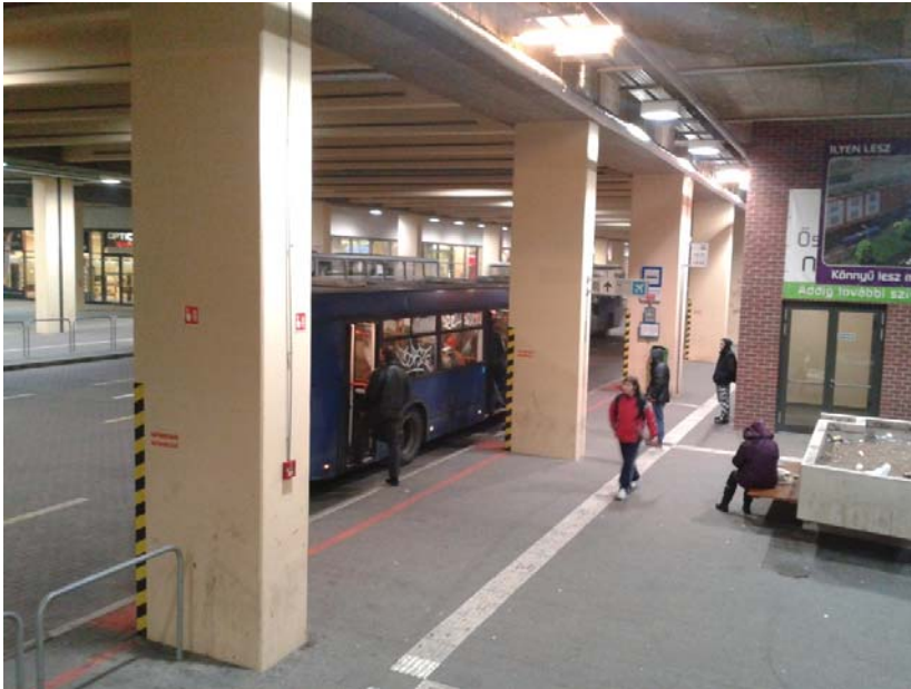
Figure 19: Example of design faults
