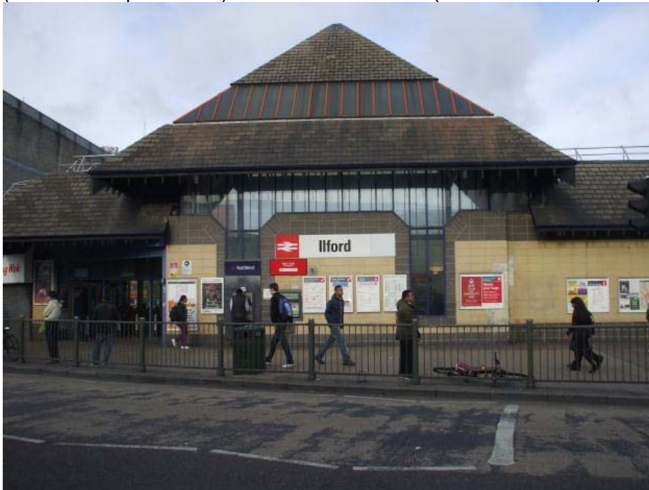
Figure 4: Main Entrance on Cranbrook Road
