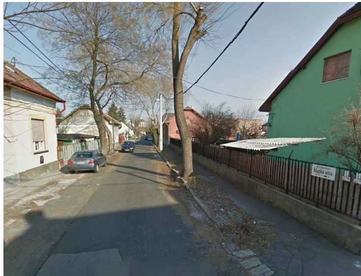
Fig. 7: Detached houses in Kispest (Source: Google Street View)
