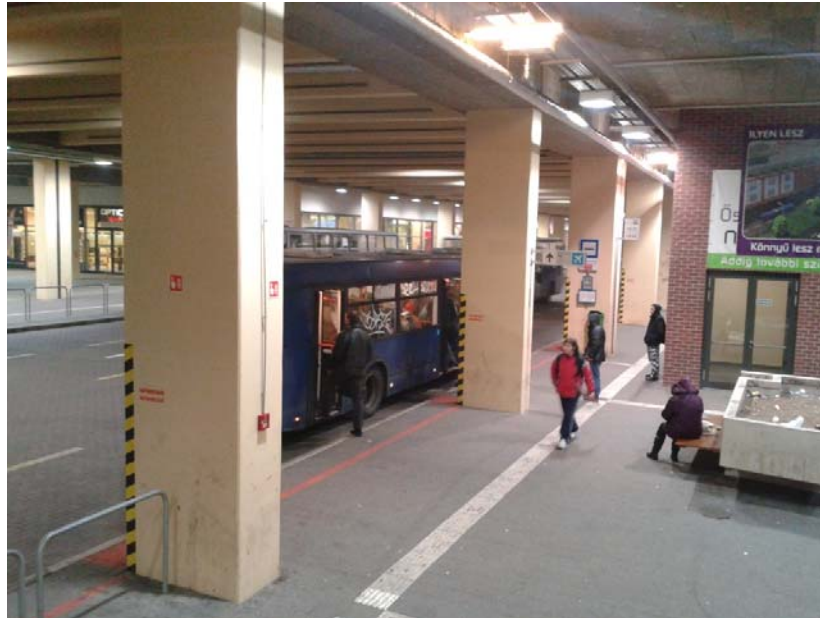
Fig. 9: Columns along the bus stops at the bus terminal
