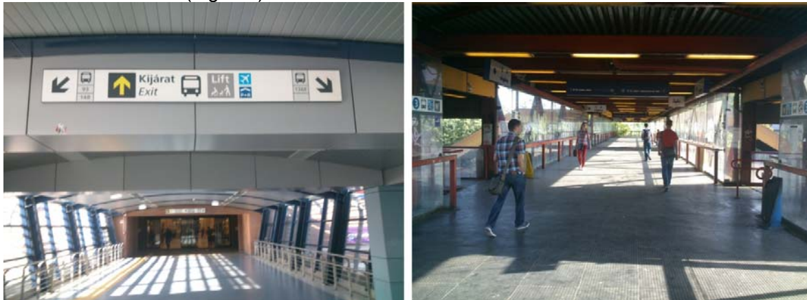
Fig. 14: The new (left) and the old (right) part of the overpass
