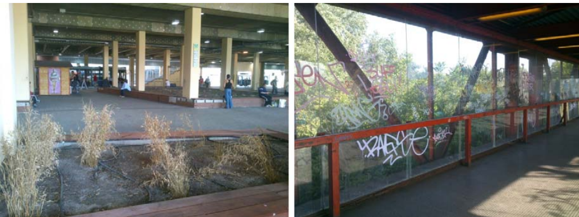
Figure 17: Lack of maintenance at Kőbánya-Kispest
