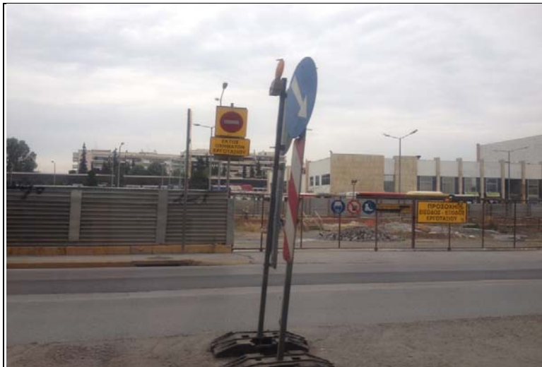
Figure 6: The under construction metro station
