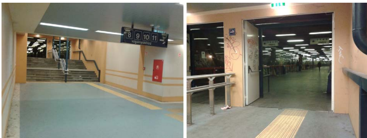
Fig. 29: End of the refurbished part of the terminal with non-accessible stairs
