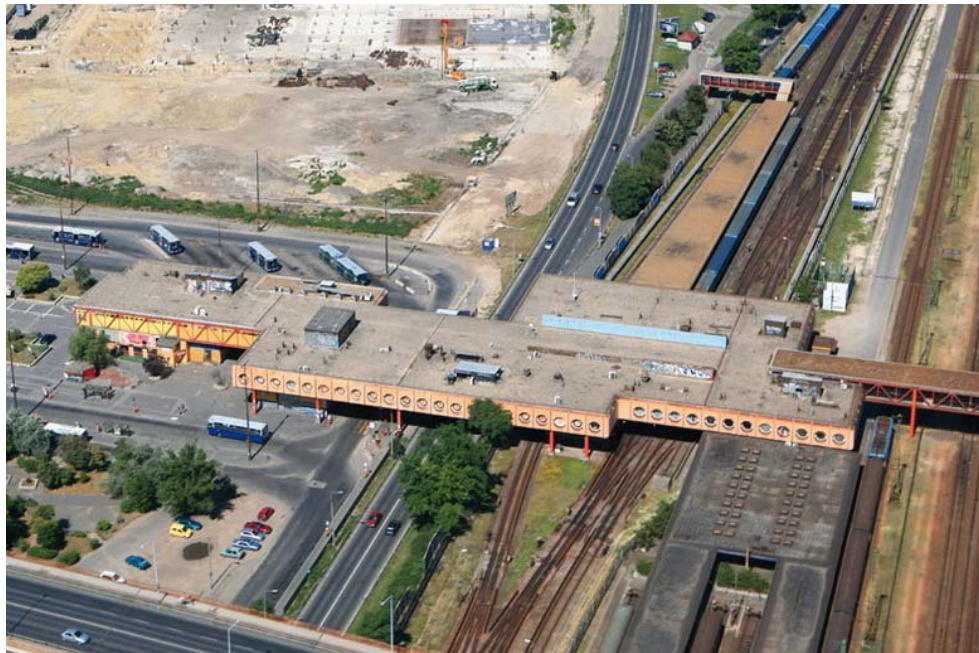
Fig. 2: Aerial view of the terminal before the refurbishment (source: http://www.globalplaza.hu/hir/oktober-14-en-nyit-a-koki-terminal )
