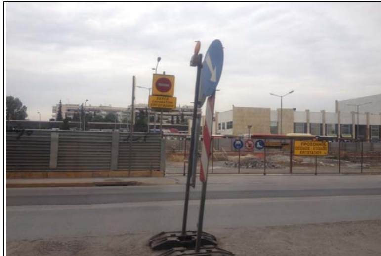
Figure 24: The under construction metro station
