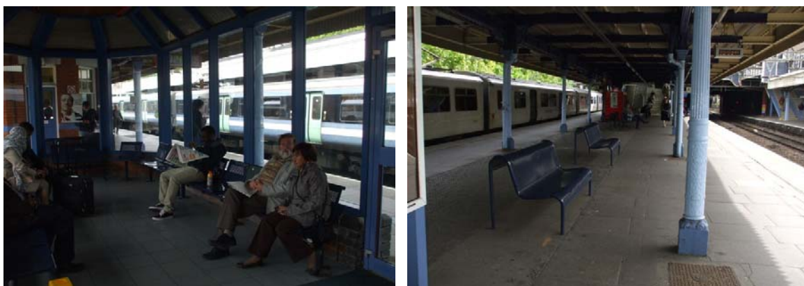
One of the waiting rooms on platform 2/3 and seating on platform 4/5.
