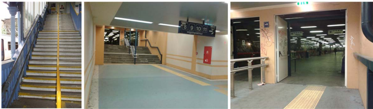
Figure 20: Examples of bad accessibility
