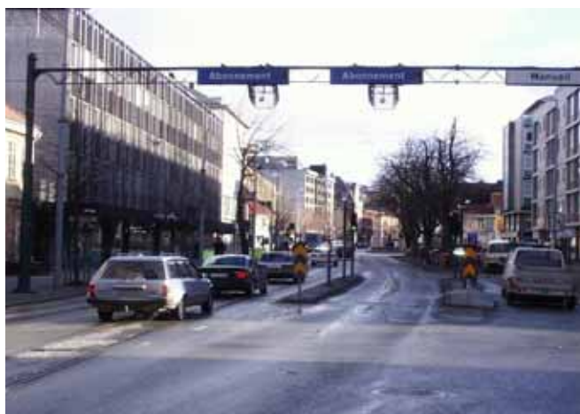
Figure 5.6 A toll plaza with two Q-FREE lanes and a manual lane in Trondheim
