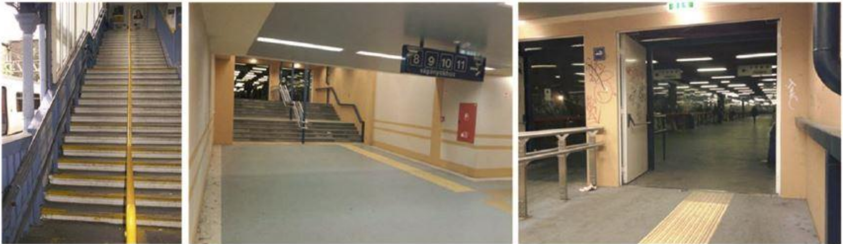
Figure 20: Examples of bad accessibility
