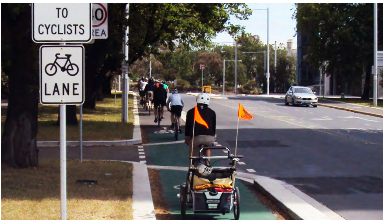
Civic Cycle Loop provides a bicycle lane that is fully separated from both motor vehicles and pedestrians in the inner city of Canberra. Photo courtesy Tony Arnold.
