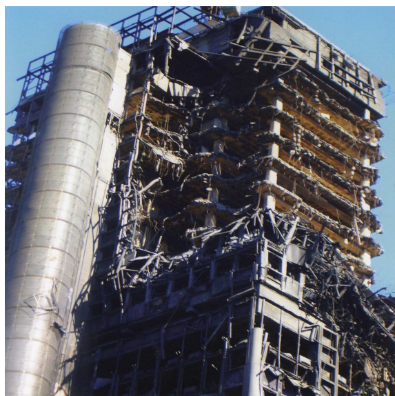
Madrid Torre Windsor fire, 2005.02.15
